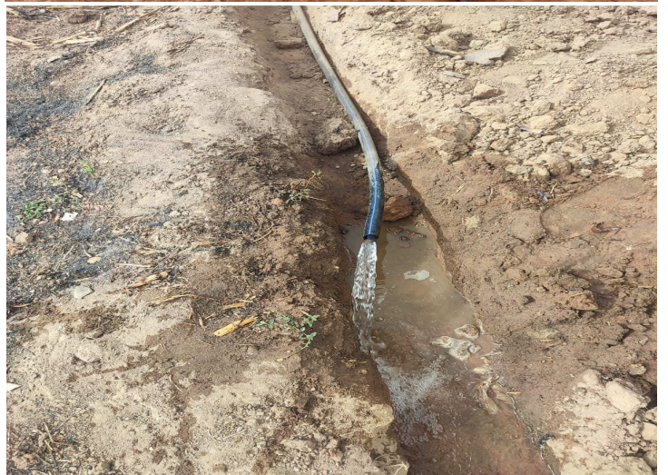
Pics: 200m digging and laying of pipe works from WASCAL borehole to MBB House
